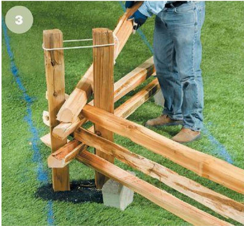
3 Install split fence rails in alternating courses at each post pair, keeping the overhangs even.
